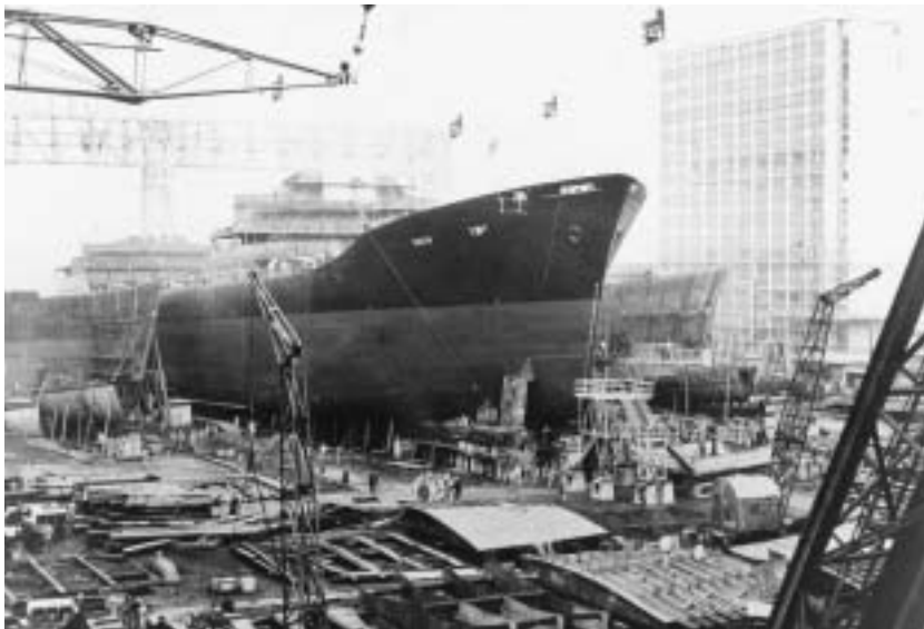
The freighter "Yafo" being built for the Israeli shipping company Zim in the German shipyards of Hamburg under the Reparations Agreement, August 1955. Courtesy of the Israel Government Press Office
